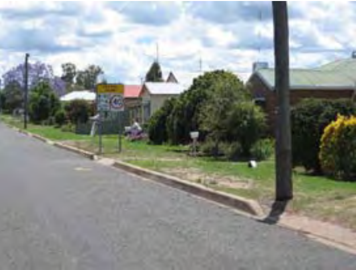
Smart Urban Design: Retention of existing trees and generous planting in front setbacks makes a positive contribution to the streetscape.
